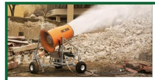
Dust control measures include wetting material prior to and during active demolition using 2" hoses connected to fire hydrants. 'Dust Boss' atomized misters (see photo) will be strategically placed on site to reduce dust and located to work with the daily wind direction.
